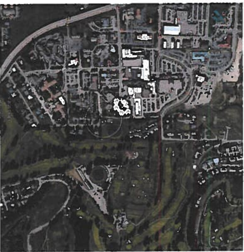
KALLSPELL, MT WATER TOWER AERIAL VIEW
